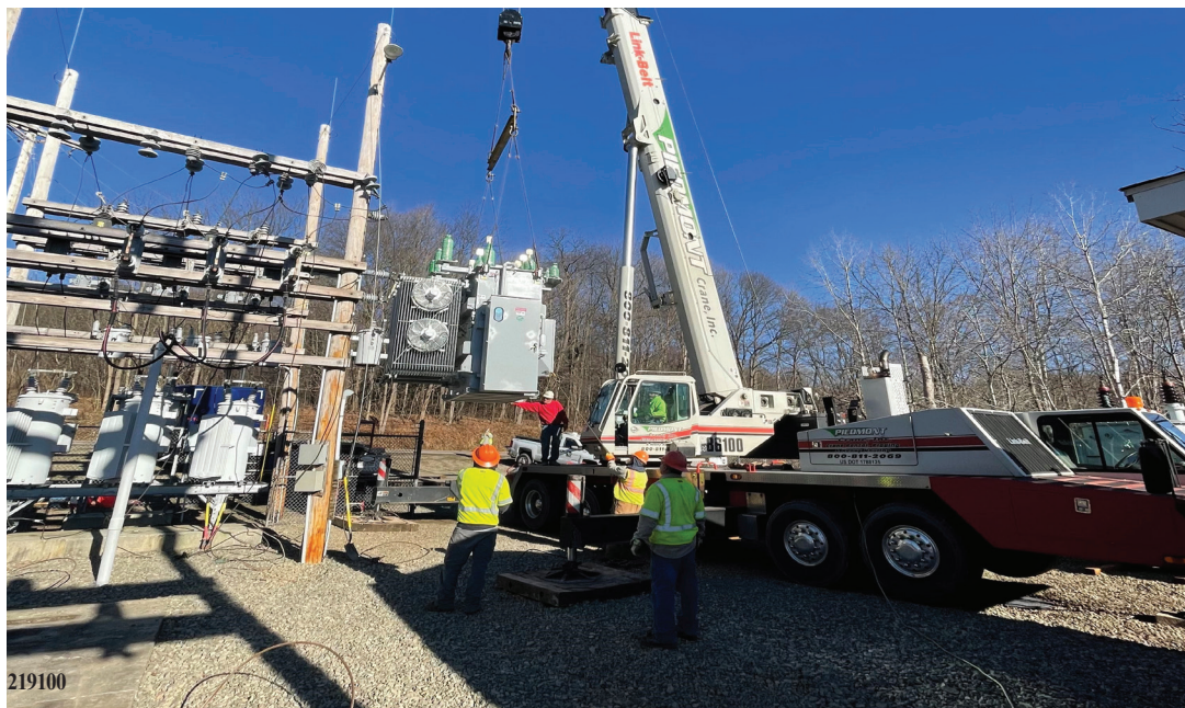
Cherry Creek linemen setting a new transformer in the Conewango Substation.
